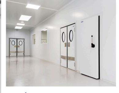
he high quality non-continuous refrigerator panel is designed for installations that require a superior sanitary finish. It has a tongue-
